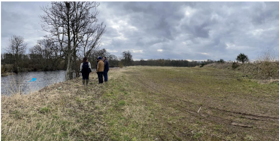
Figure 12. Example where the flood embankment is set back up to 60m from the riverbank allowing space for natural river processes and flood conveyance and avoiding any beaver burrowing activity due to the distance from the river bank. The grassed area could be improved by encouraging mixed vegetation growth.
