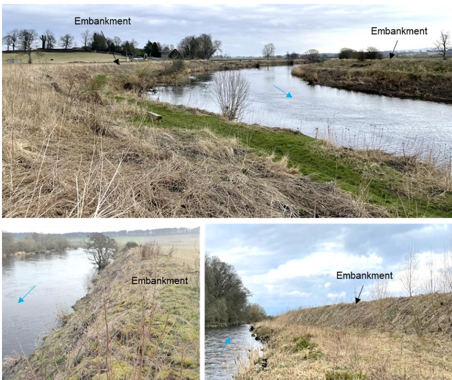
Figure 6. Photos showing embankments on the River Isla taken in March 2022, blue arrows indicate flow direction. Embankments are commonly set back a short 2-10m distance from the water edge (top photo and bottom right photo) or located directly on the bank top (bottom left photo).
